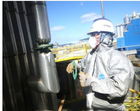
SEAL AIR BALANCE 작업
